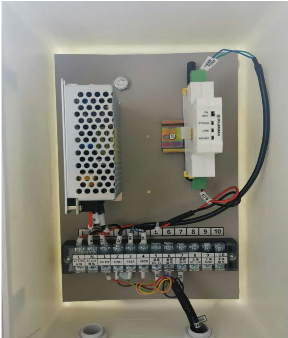
Wiring Finished display
